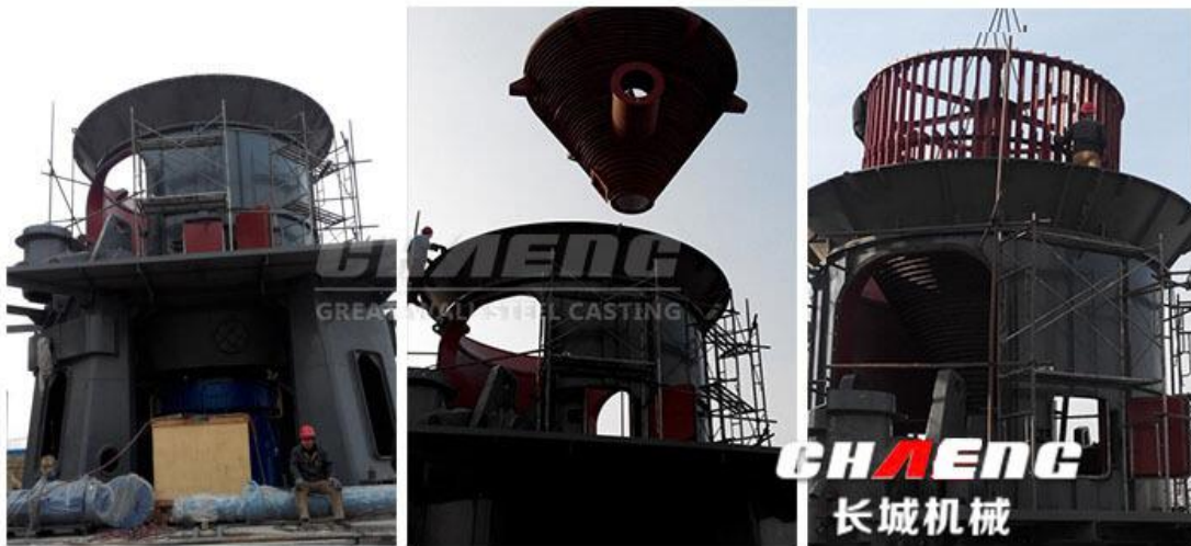
Shanghai Baosteel slag vertical mill separator installation picture
